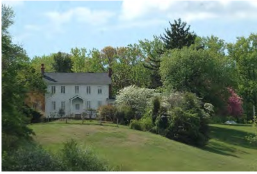
The historic home and office of the Alice Ferguson Foundation.
