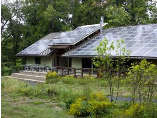
The Cafritz Environmental Center of the Alice Ferguson Foundation, one of the greenest buildings in the world, received full certification under the Living Building Challenge™ by the International Living Future Institute. Photos: Alice Ferguson Foundation.
